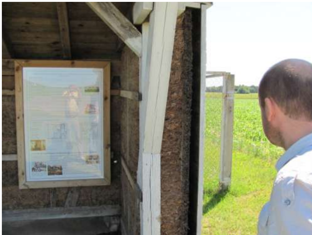
Demo Model and description of one of construction technology: wood-chips-clay wall with reed mesh.
