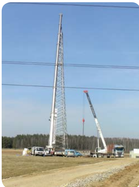
Construction of Smalininkai power plant's hub (Photographer Gintaras Nenorta)
