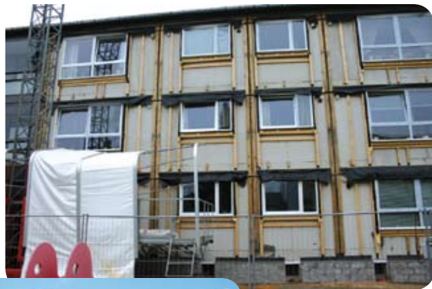
Building under renovation (Photographer Soren Dyck-Madsen)
