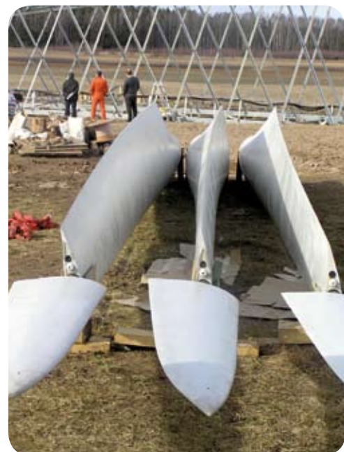
Blades of wind turbine waiting for the assembling (Photographer Gintaras Nenorta)
