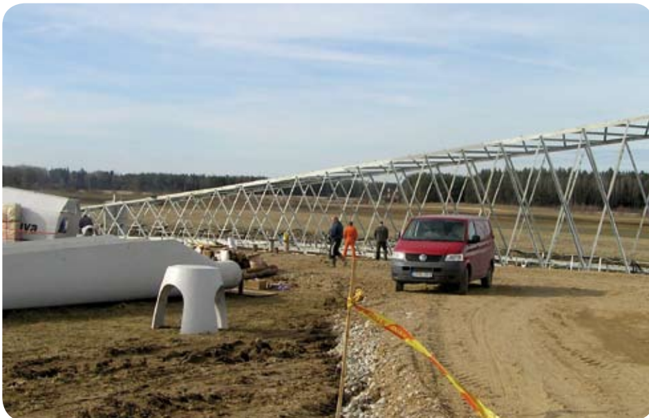
Wind plant construction site (Photographer Gintaras Nenorta)
