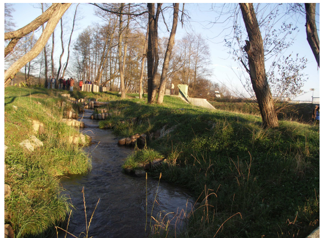
Fig. 2. Dam bypass to free fish migration.
