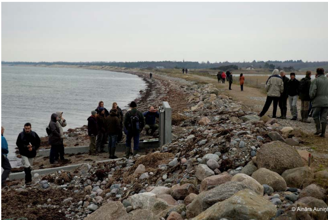
Fig.4. Dam and sluice built in project IMAGE to stabilize hydrological condition in coastal lagoon.
