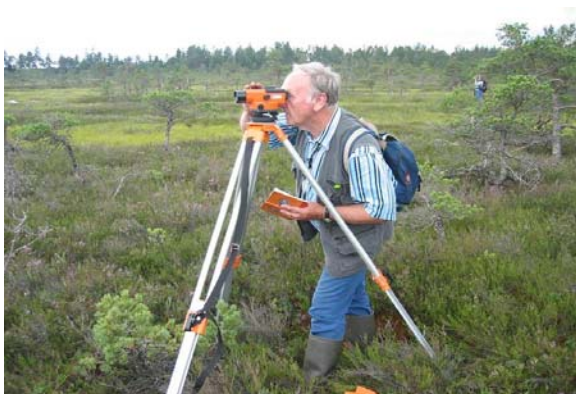
Levelling of Vasenieku Mire for building of nature trail (Photo by Mara Pakalne)
